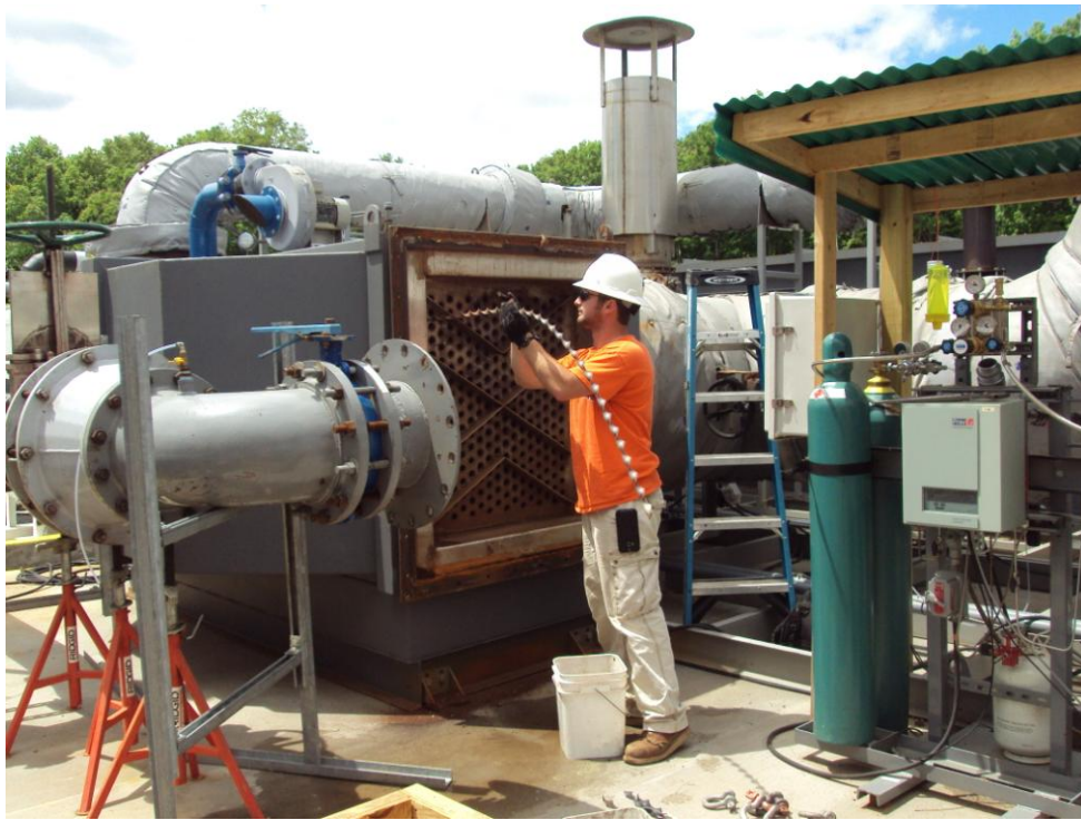
Date: 5/5/14 TerraTherm installing turbulators to increase efficiency of the oxidizer.
