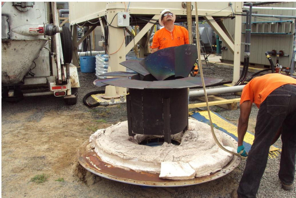
Date: 8/21/2014 View of damaged daisy wheel.
