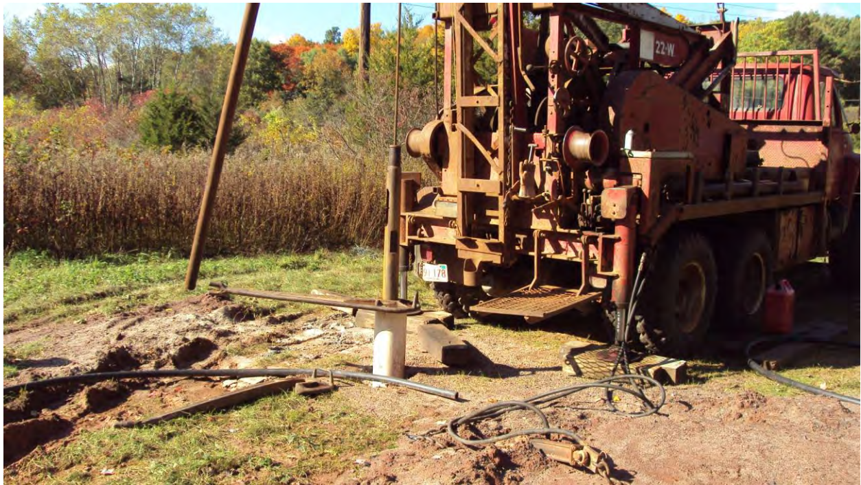
Date: 10/17/2014 Completing installation of recovery well RW-15.
