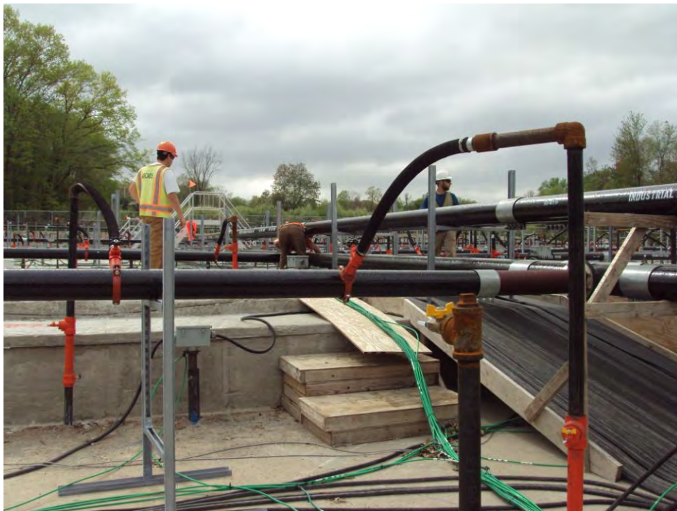
Date: 5/15/2014 Orientation: East looking West Starting Phase 1 operation of the ISTR system, vapor extraction wellheads are being adjusted to maximize and equalize flow across the wellfield and the wellfield piping is being inspected for air leaks.
