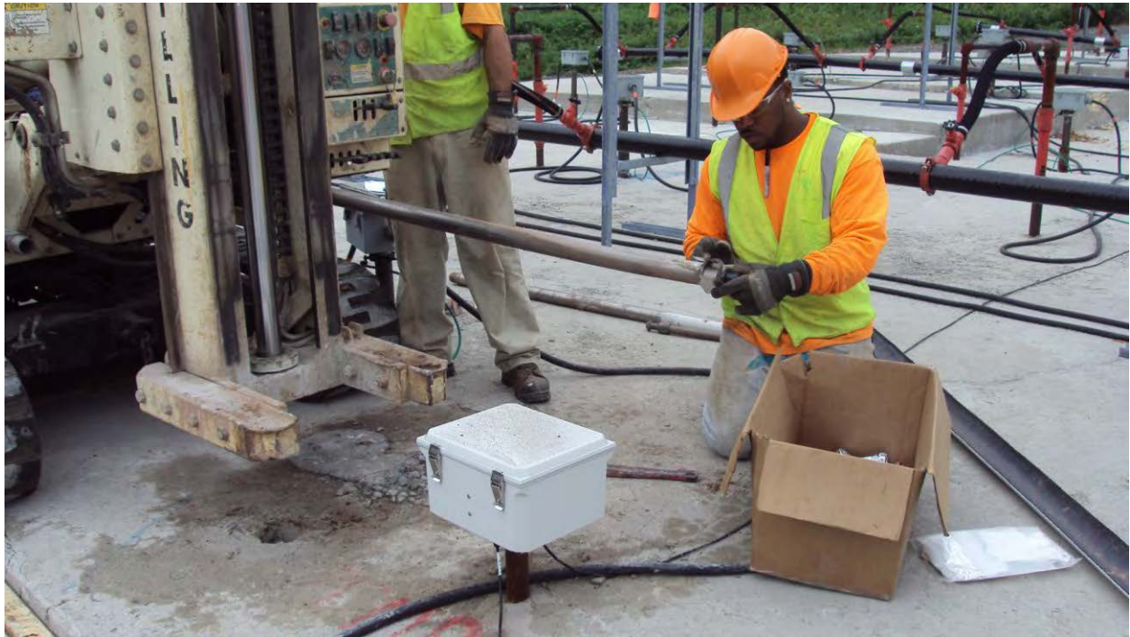
Date: 10/13/2014 Preparing to extract soil sample during Phase I interim sampling.
