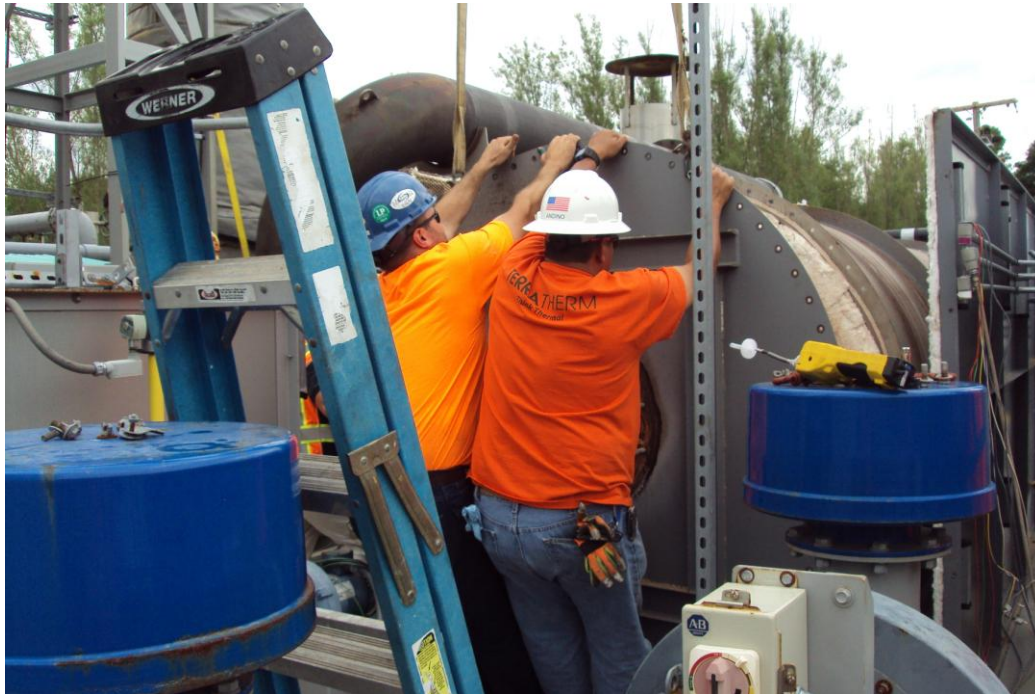
Date: 8/12/2014 TerraTherm disassembling oxidizer and removing daisy wheel.
