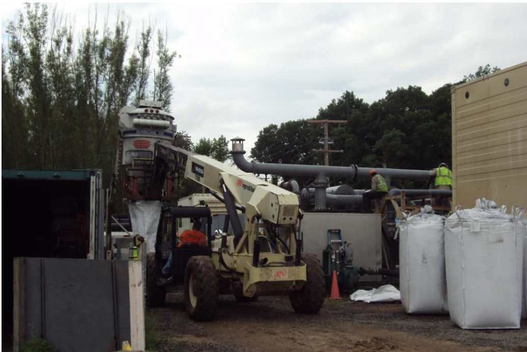
Date: 8/22/2014 View of carbon change out being performed.
