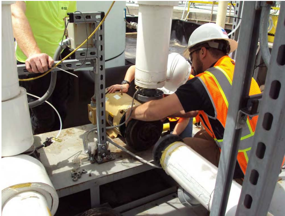
Date: 5/7/2014 Repairing scrubber pump unit.
