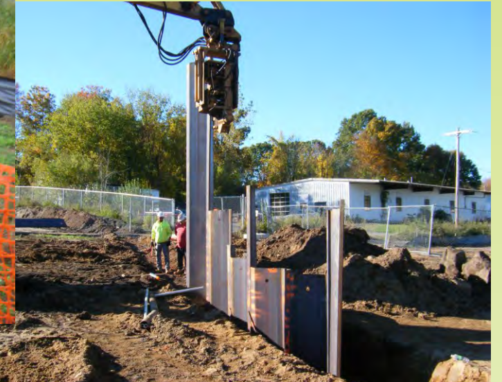
Installing the extension to the barrier wall around the treatment zone.
