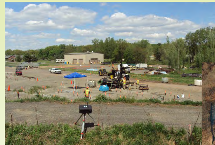
Installing vapor extraction wells for the thermal treatment process.
