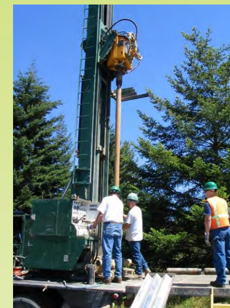
Drilling a groundwater monitoring well
