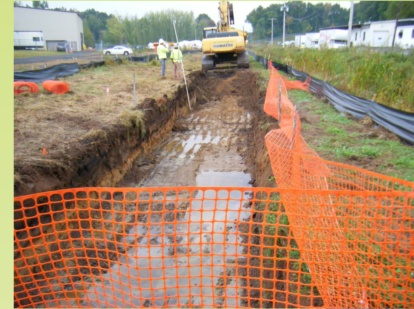
Left: Excavating along the northern end of the railroad tracks. Below: Installing the extension to the barrier wall around the treatment zone.
