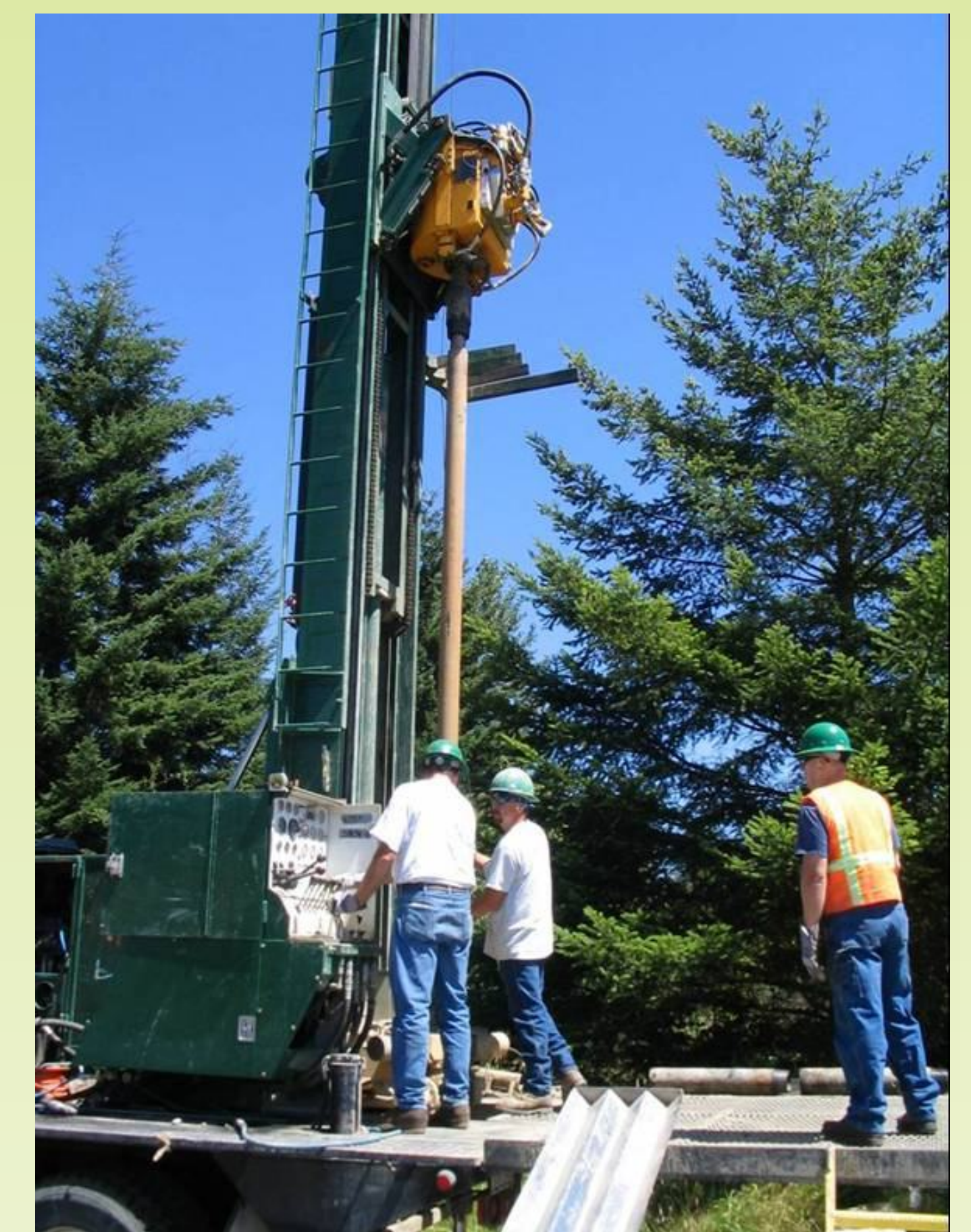
Drilling a groundwater monitoring well
