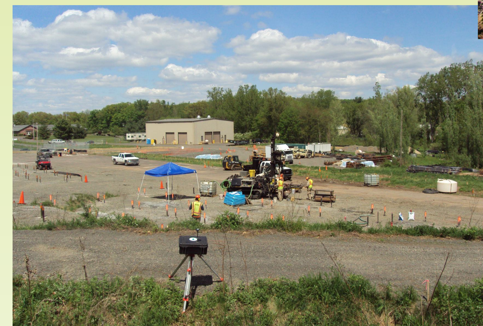
Left: Installing vapor extraction wells for the thermal treatment process. Below: View of the former Operations Area in December 2010 after completion of grading work.
