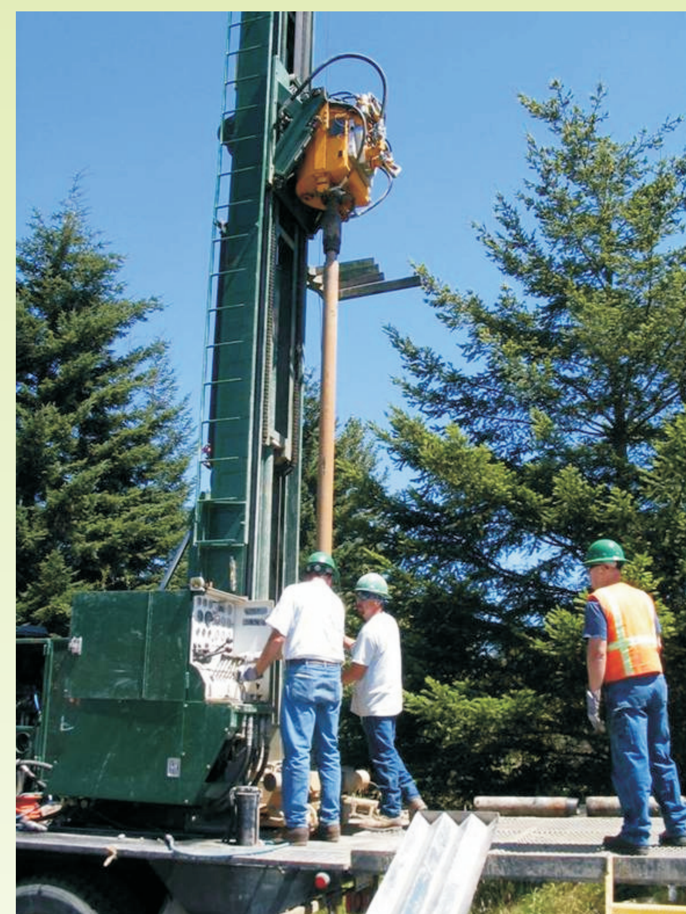
Drilling a groundwater monitoring well
